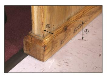
If the pew supports have wider bases (not flush with the support), measure the height of the base <sup>(4)</sup> as well as the width it extends out from the support. <sup>(5)</sup>
