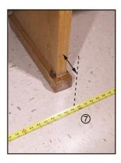
If the back of the middle support does not extend as far out as the end supports, measure how much it is set in. To do this, stretch a measuring tape or other long straight edge from one end support to the other end support. Then measure the distance from the back of the middle support to the straight edge.
